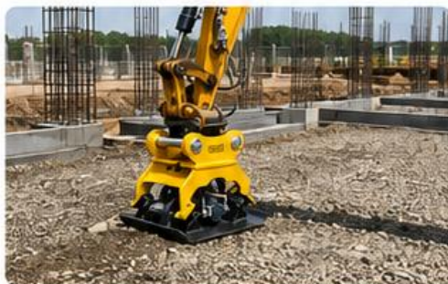
4. Foundation Compaction
