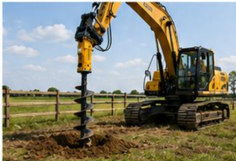
1. Fence Post Drilling
