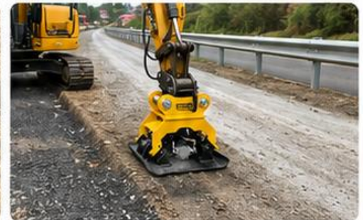
3. Road Edge Work
