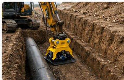
5. Pipeline Backfill
