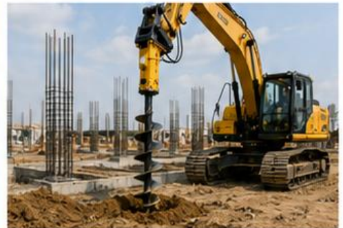
3. Foundation Drilling
