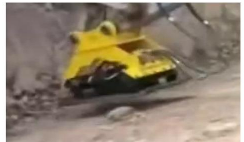
3. Road Edge Work
