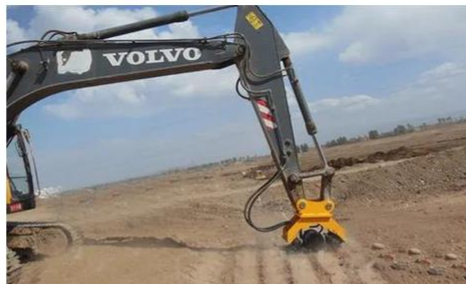
2. Slope Compaction
