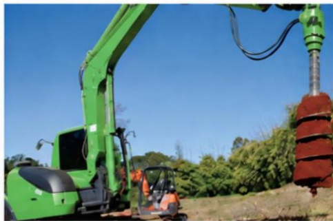
4. Pole Installation
