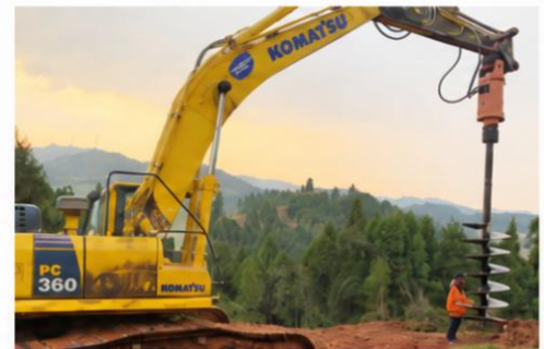
3. Foundation Drilling
