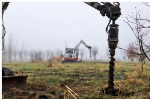
1. Fence Post Drilling
